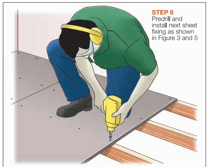
FIGURE 11 PRE DRILL NEXT SHEET
